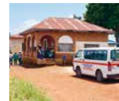
Partner sein constructed this medical centre | K 14
